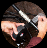
Moist and Corrosive Environments
