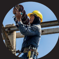
Moist and Corrosive Environments
