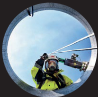
Outdoor or Underground
